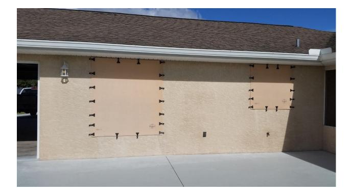
In the above application, both window attachment spans are side to side and the two additional anchors top and bottom, although not required, were desired by the homeowner. In this application, the order will provide for the required 24 Clips and anchors on the sides. The optional supplemental anchors (4 or 8) should be added to your order.
